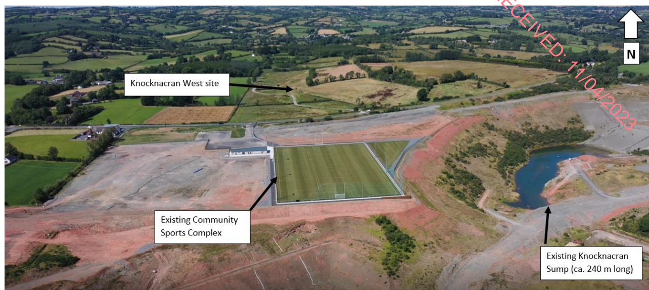
Figure 8.26: Aerial photo showing the existing Knocknacran sump on the site, the size is variable, but it is currently ca. 240 m long
