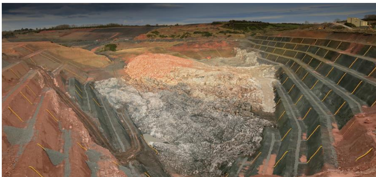
Figure 8.27: Good surface runoff management practices at the Knocknacran Open-Cast, including plating of the bench faces and drainage of the benches
